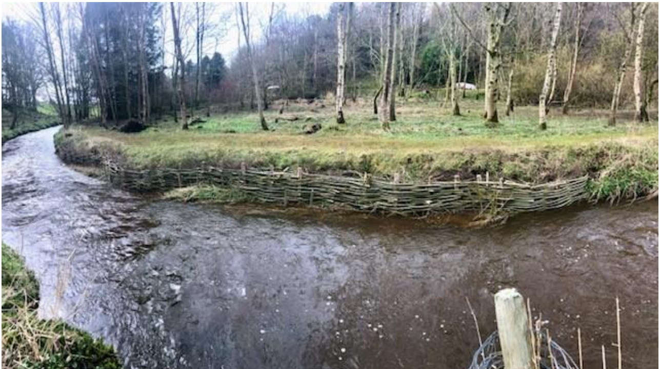
Ebrie Willow Bank Repair April 2022.
