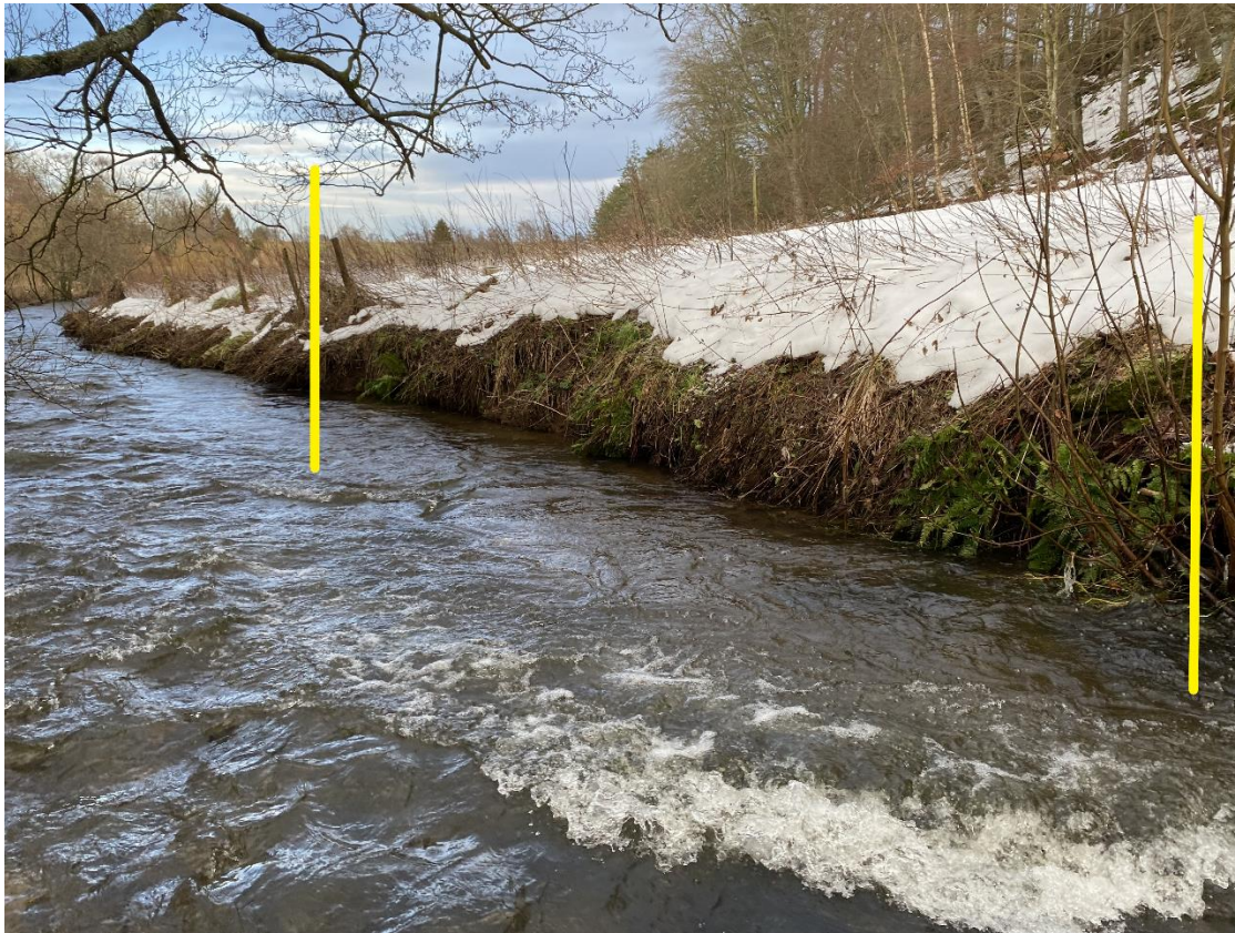
Fig 4, Below Fourdon burn bank erosion site, between the yellow lines.
