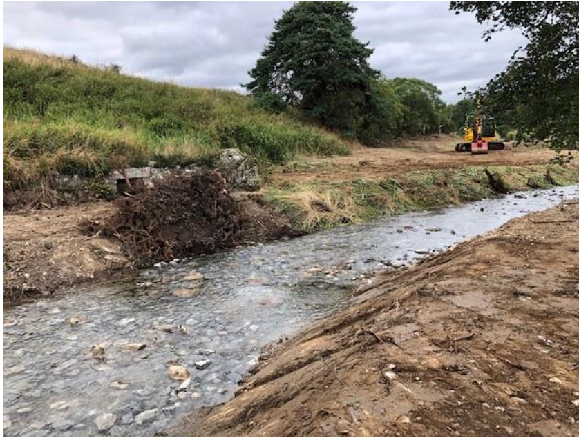
Fig 2, A meander has been added to the section upstream of the weir.
