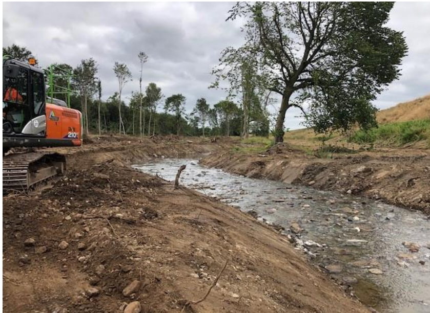
Fig 2, A meander has been added to the section upstream of the weir.
