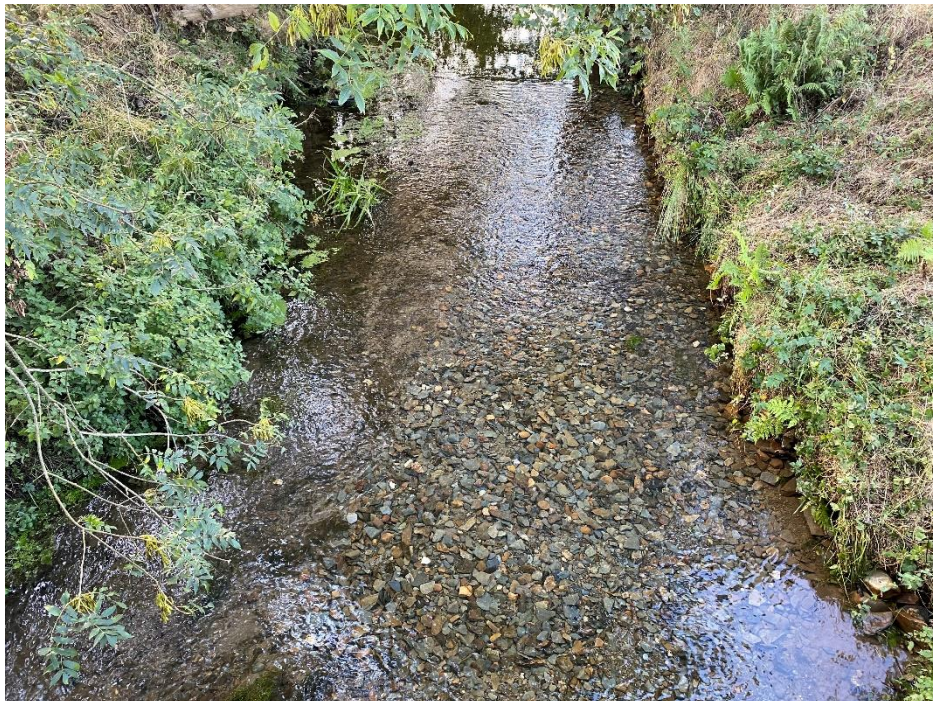
Fig 6, Completed section now cleaned, the water flow is now flowing through the gravel and not just flowing over. Now the river flow is flowing through the gravel, this will increase oxygen levels within the substrate for the forthcoming spawning season and promote better survival from egg to emerging fry.
