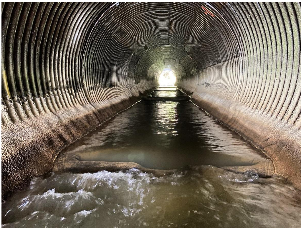
Fig 1, Series of 4 Pre-weirs within the Culvert
