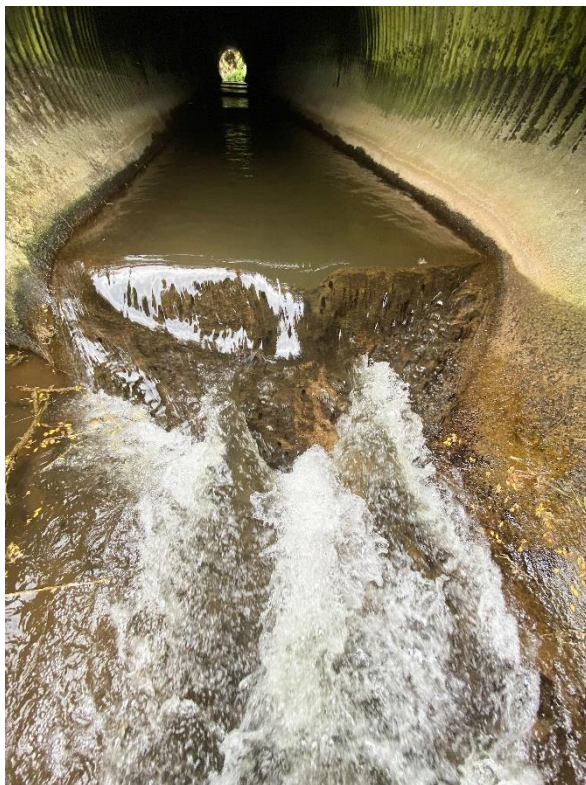
Fig 2 upstream view of high step before entering the Culvert.
