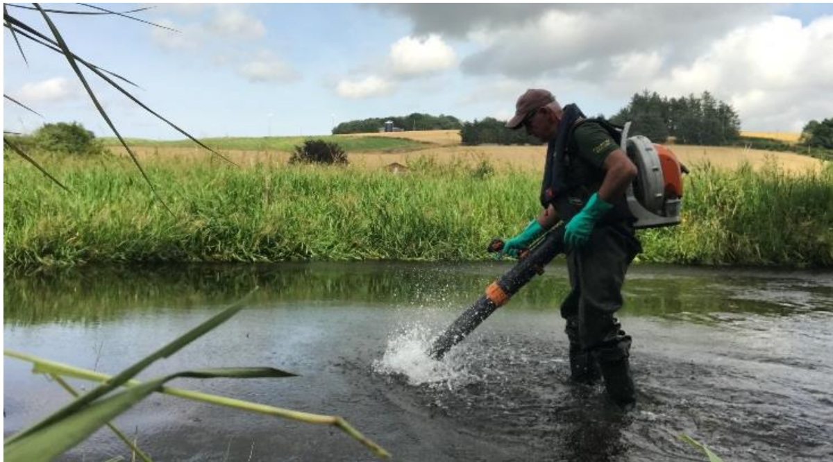
Figure 10. Leaf blower being used for cleaning the spawning gravel.
