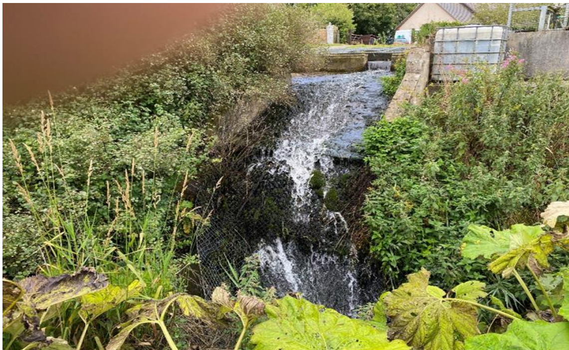
Fig 4, Spillway from hydro scheme.
